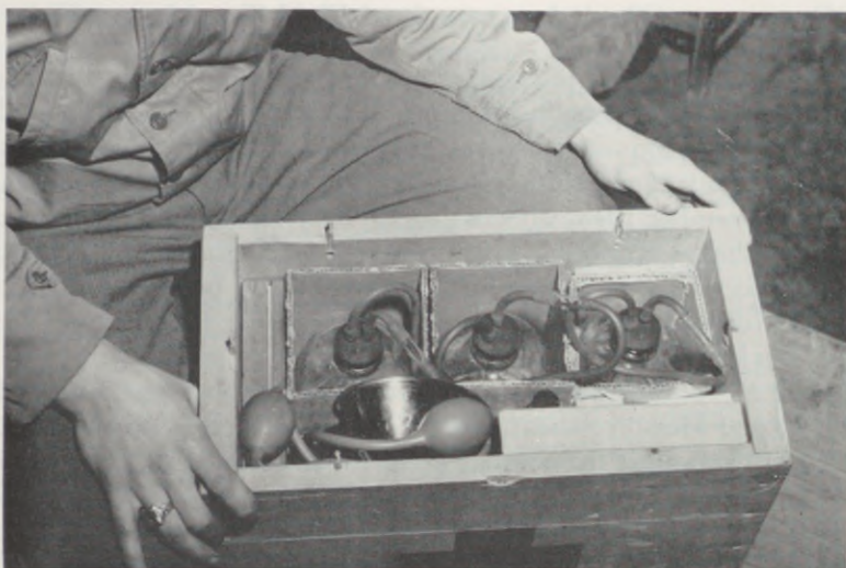
FIGURE 51.—Ebert-Emerson transfusion set, packed in ammunition box and ready for use. Each box contained three transfusion bottles and accessory equipment.
